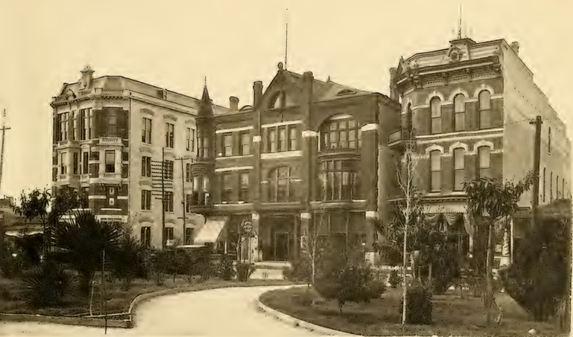
OPERA HOUSE AND MEXICAN CONSULATE—ALAMO PLAZA.
